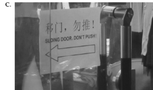
FIGURE 1.3. Sliding Doors: Seldom Done Well. Sliding doors are seldom signified properly. The top two photographs show the sliding door to the toilet on an Amtrak train in the United States. The handle clearly signifies “pull,” but in fact, it needs to be rotated and the door slid to the right. The owner of the store in Shanghai, China, Photo C, solved the problem with a sign. “DON’T PUSH!” it says, in both English and Chinese. Amtrak’s toilet door could have used a similar kind of sign. (Photographs by the author.)
