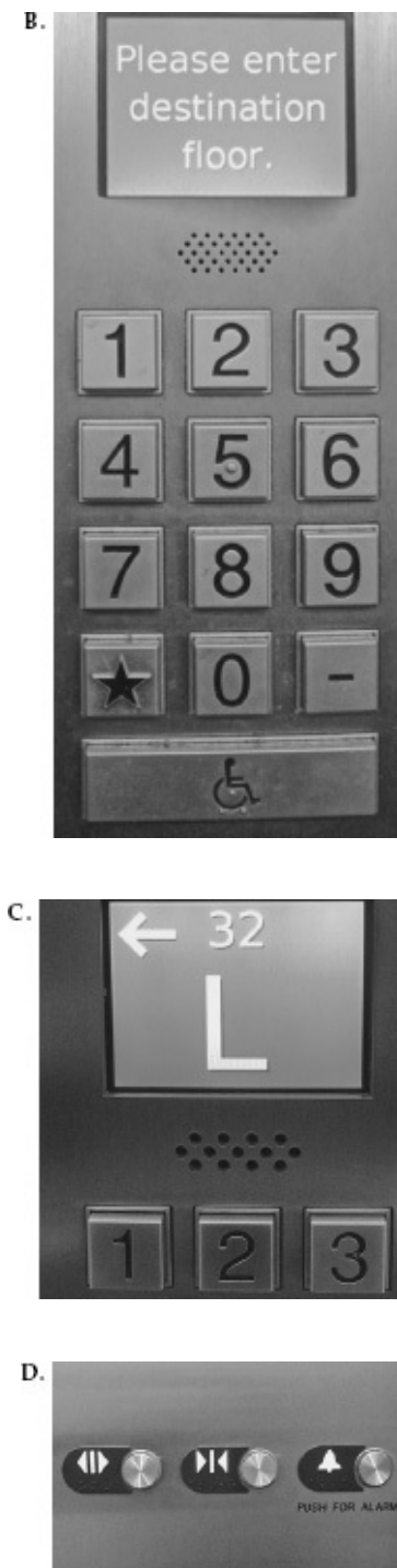
FIGURE 4.8. Destination-Control Elevators. In a destination-control system, the desired destination floor is entered into the control panel outside the elevators (A and B). After entering the destination floor into B, the display directs the traveler to the appropriate elevator, as shown in C, where “32” has been entered as the desired floor destination, and the person is directed to elevator “L” (the first elevator on the left, in A). There is no way to specify the floor from inside the elevator: Inside, the controls are only to open and shut the doors and an alarm (D). This is a much more efficient design, but confusing to people used to the more conventional system. (Photographs by the author.)
